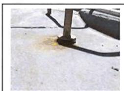
Hand rail rusted out.
