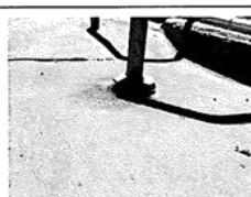
Hand rail rusted out.
