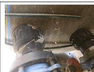
Leaking seal on Sand filter.
