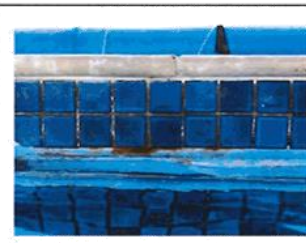
Rust coming through at the shallow end of 25m pool
