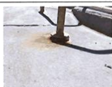
Hand rail rusted out.
