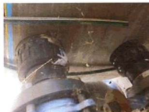
Leaking seal on Sand filter.
