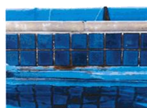
Rust coming through at the shallow end of 25m pool
