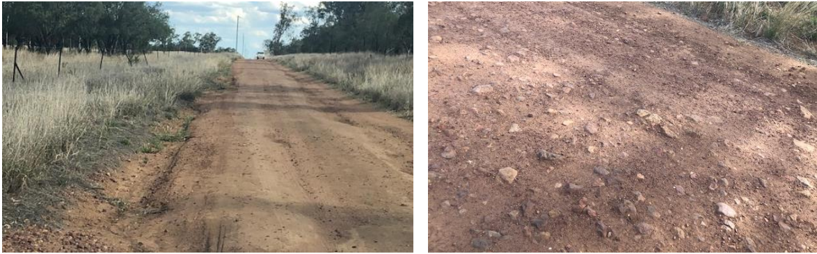
Figure 9 – Ch 1.000 of the unnamed roadway – Off Blue Hills Road – Water ponding area
