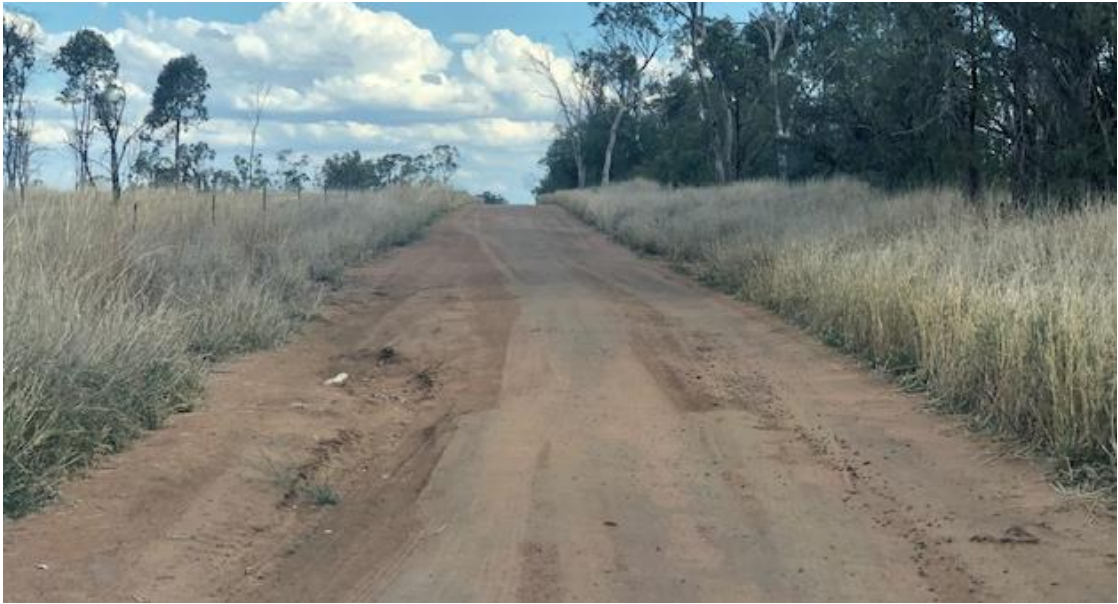
Figure 6 – Ch 300 of the unnamed roadway – Off Blue Hills Road – Scour
