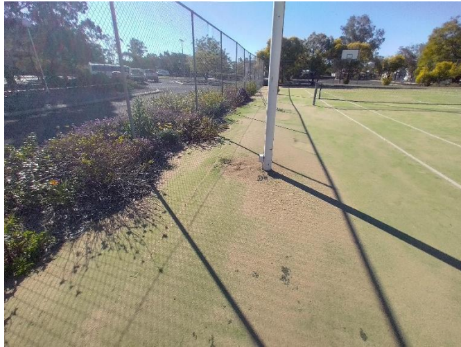
Figure 6 - pits and hollows on Court 8 due to deterioration of court base substrate
