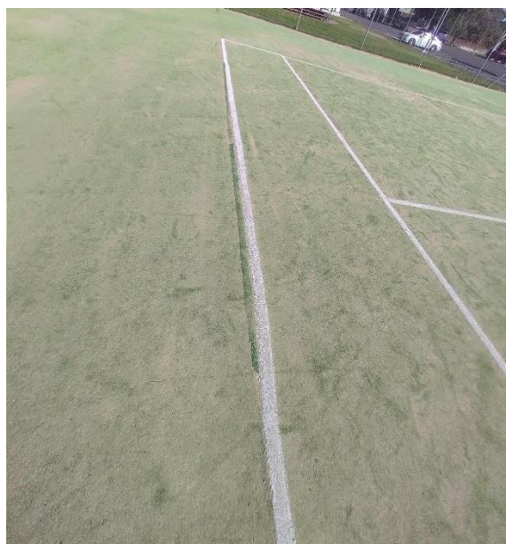
Figure 3 - Wear and tear of synthetic court
