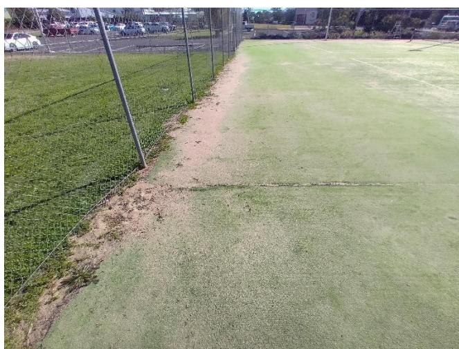
Figure 5 - Wear and hollow on court 7 due to compromised base formation underneath the court
