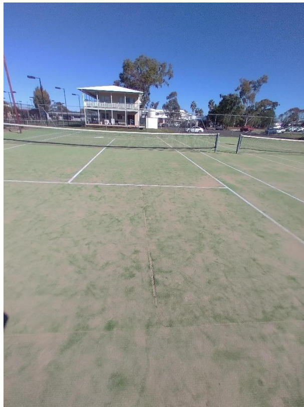
Figure 2 - Partial replacement of synthetic surface and subsequent deterioration of join
