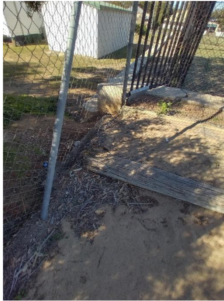
Figure 9 - Deterioration of fence and log retaining wall on court 7
