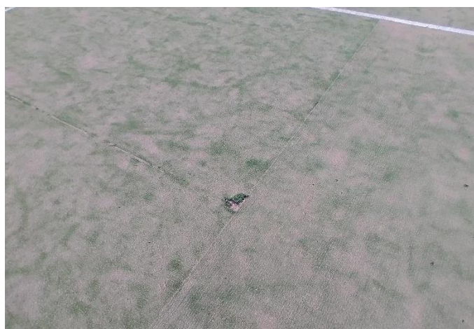
Figure 4 - Partial Replacement of synthetic surface and subsequent tear at join
