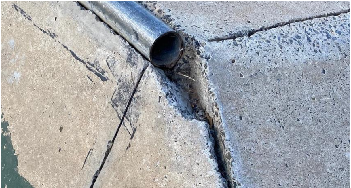
Photos 3 and 4 – damaged cement at ends of pipe
