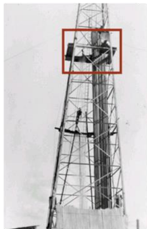
Monkeyboard where derrickman works. Note stand of pipes inside derrick
