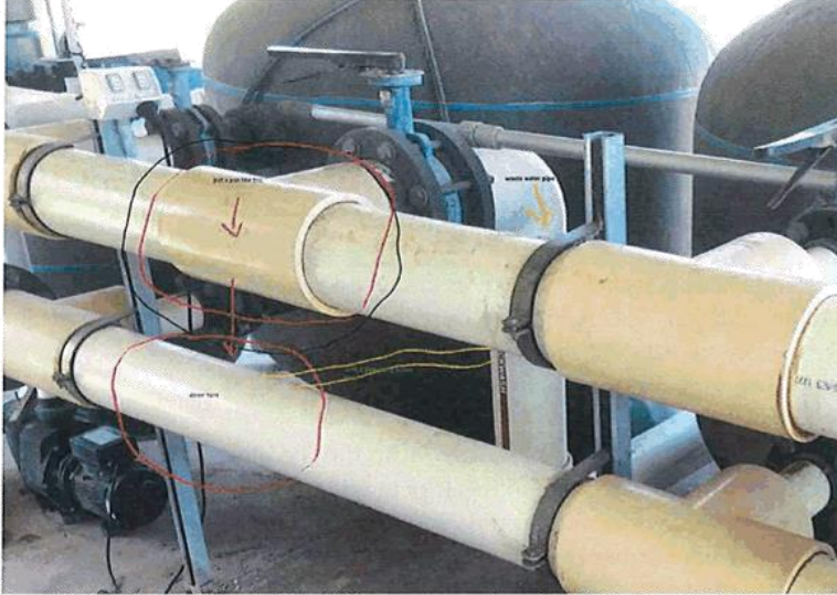
Photo above – proposed pipe work for rinse.
