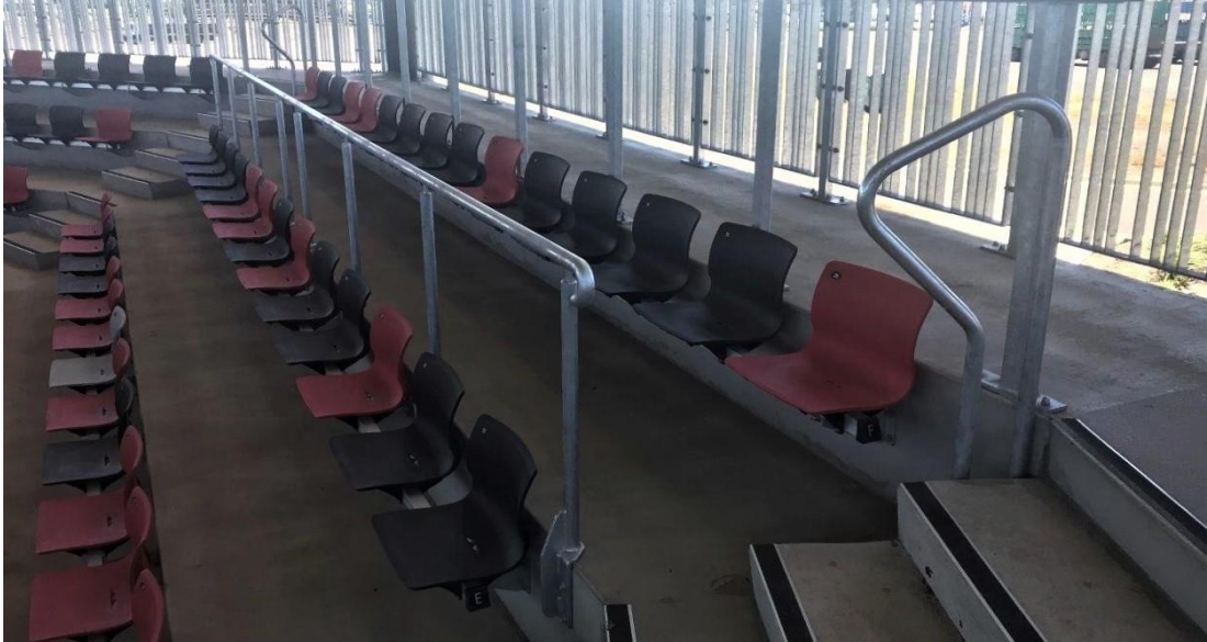
Trial Barrier Rail installed at Stud Arena
