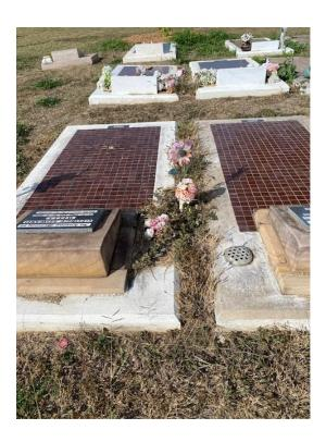
Photo showing an example of a permanent strip of concrete between graves
